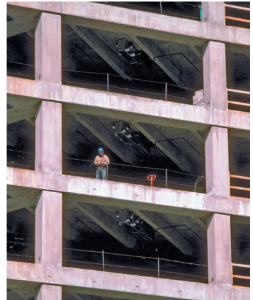
Photo 4.4 Reinforced concrete building.
