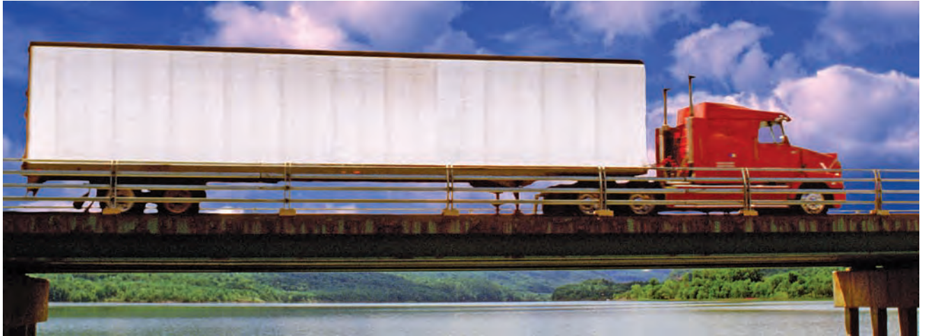
Photo 9.5 The deflections of the beams used for the bridge must be reviewed for different possible positions of the truck.
