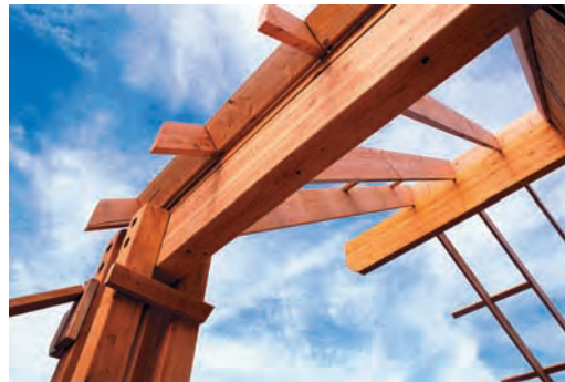
Photo 5.1 Timber beams used in residential dwelling.
